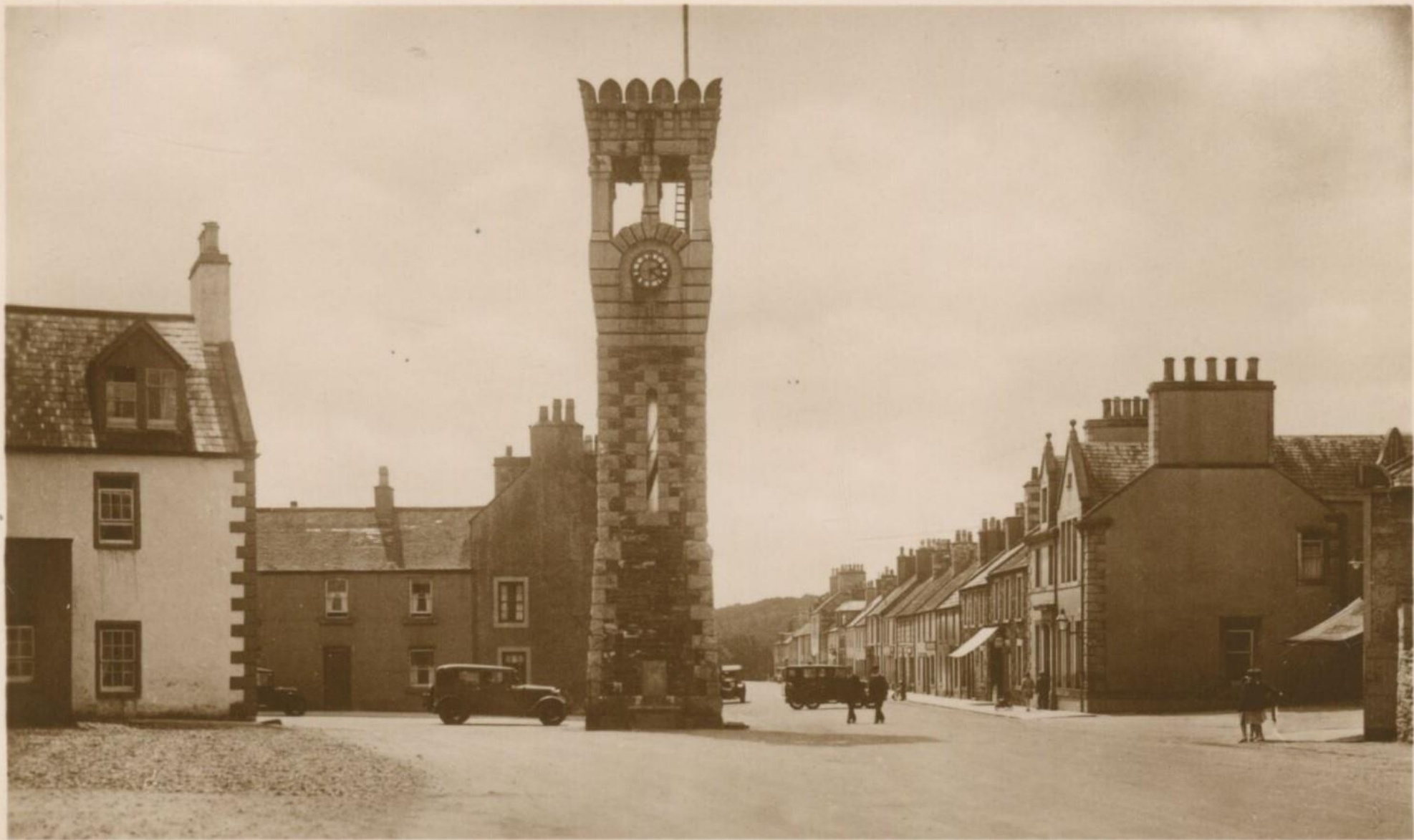
THE CLOCK TOWER, GATEHOUSE OF FLEET
